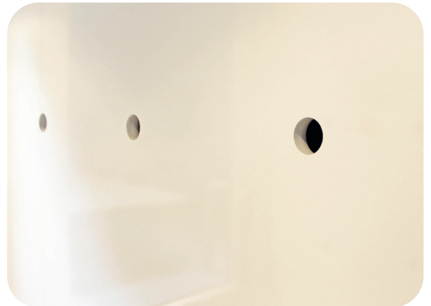
The air leaving the 30 nozzles with a diameter of 38 mm, has a velocity in excess of 100 km/h.
